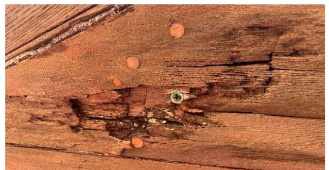
Close-up view of one area of rot.
