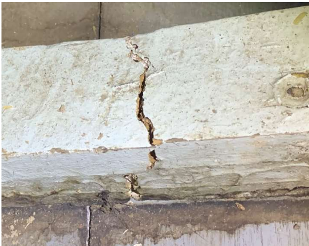
(5) Cracked Ribs need replacing
