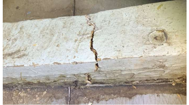
One of the cracked ribs needing replacement
