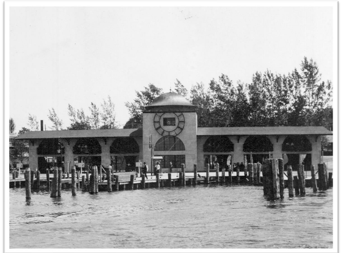
Twin Cities Rapid Transit Company's Excelsior Dock Station
